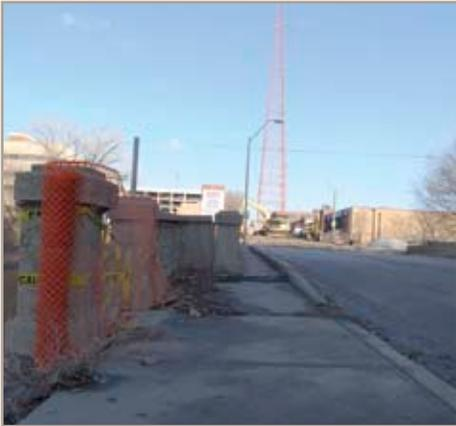
The old two-lane bridge by the Association's offices (shown here in February) is being replaced with a three-span, pre-stress girder bridge with curtain walls for the two side spans.
